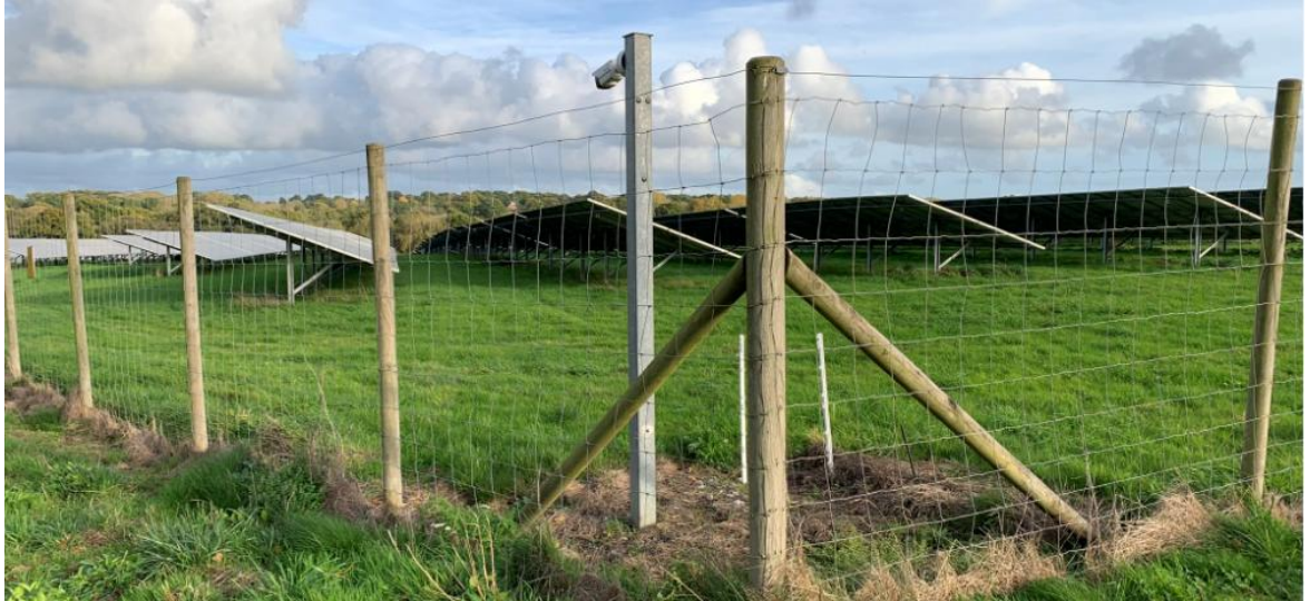
Figure 15-18: Typical Deer Fencing
