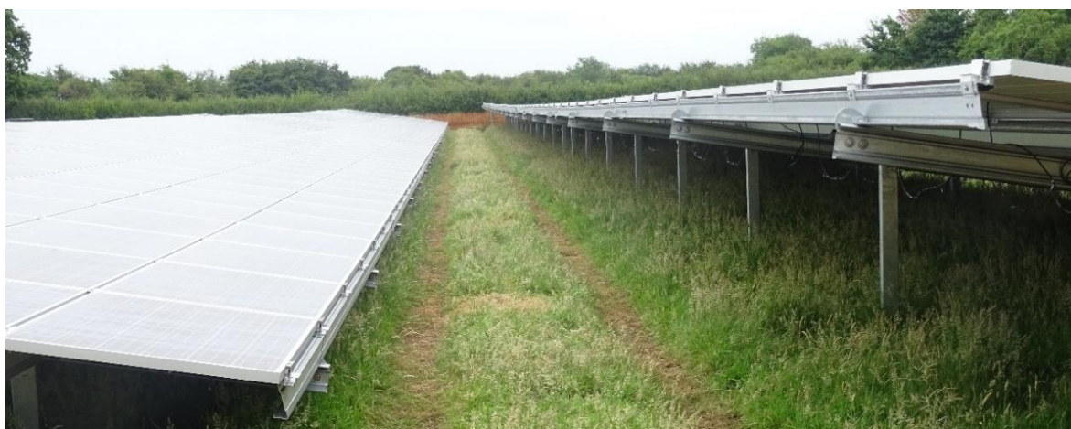
Figure 15-13 :Part Installed Panels (Bentham Farm, Purton)
