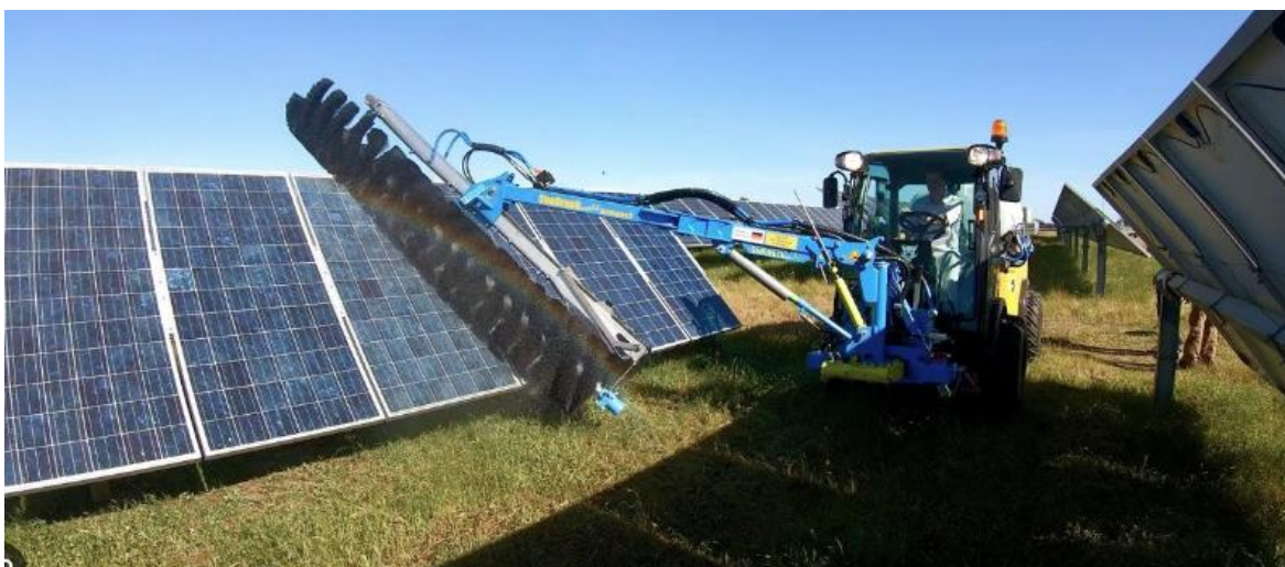
Figure 15- 20: Cleaning of Solar Modules
