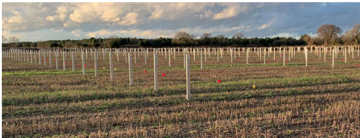
Figure 15-12 :Mounting Structure Piles being Installed (taken at Tiln Farm, Retford, in January 2023)
