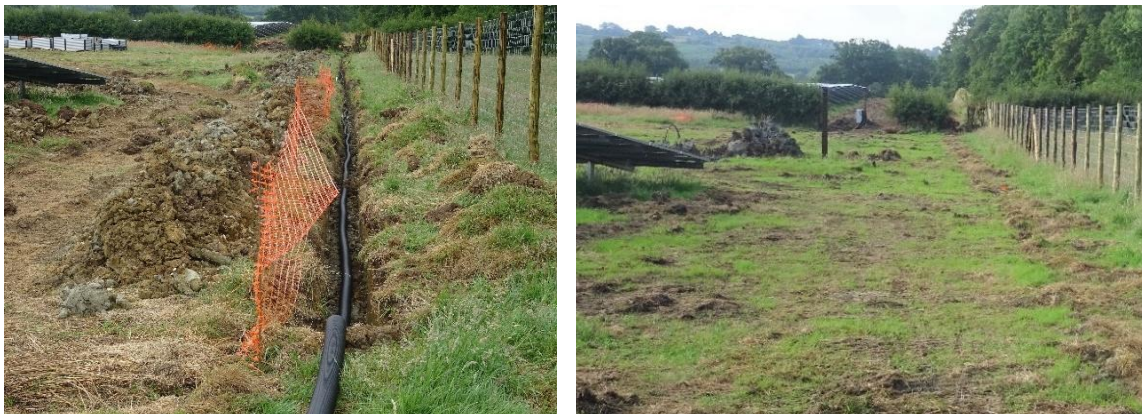
Figure 15-16: Cabling Channels during Cable Installation
