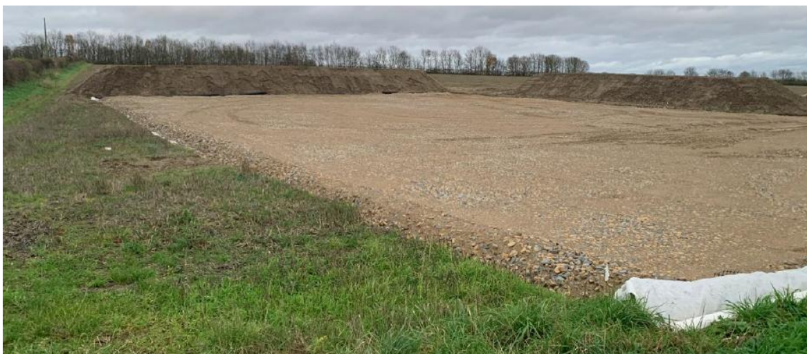
Figure 15-15 :Newly Installed Construction Compound
